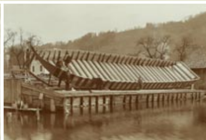
Construction of a Trauner in the shipyard of Captain Johann Kagerer in Gmunden-Weyer.
