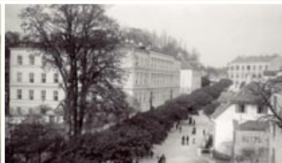
The Habertstrasse with the school building about 1905.
